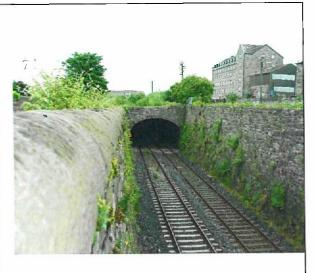
Westmoreland tunnel from the west – note the lack of parapet and the stone retaining walls flanking the railway
